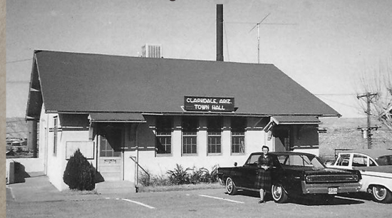
Town Hall Building 1960s - Now the Museum
